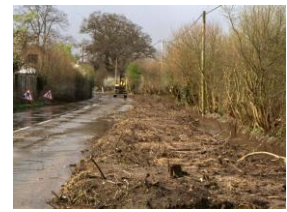
Digging out the ditch in Lower Assendon.
